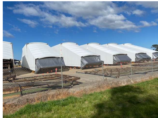
Hangar 1 trusses covered in plastic to protect them from the weather (Photo courtesy of John Phillips)
